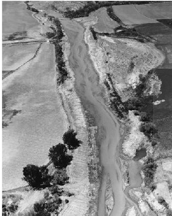
Figure 12.1. Army Corps of Engineers clearing and snagging of the Owyhee River below Owyhee Dam, 1954.
