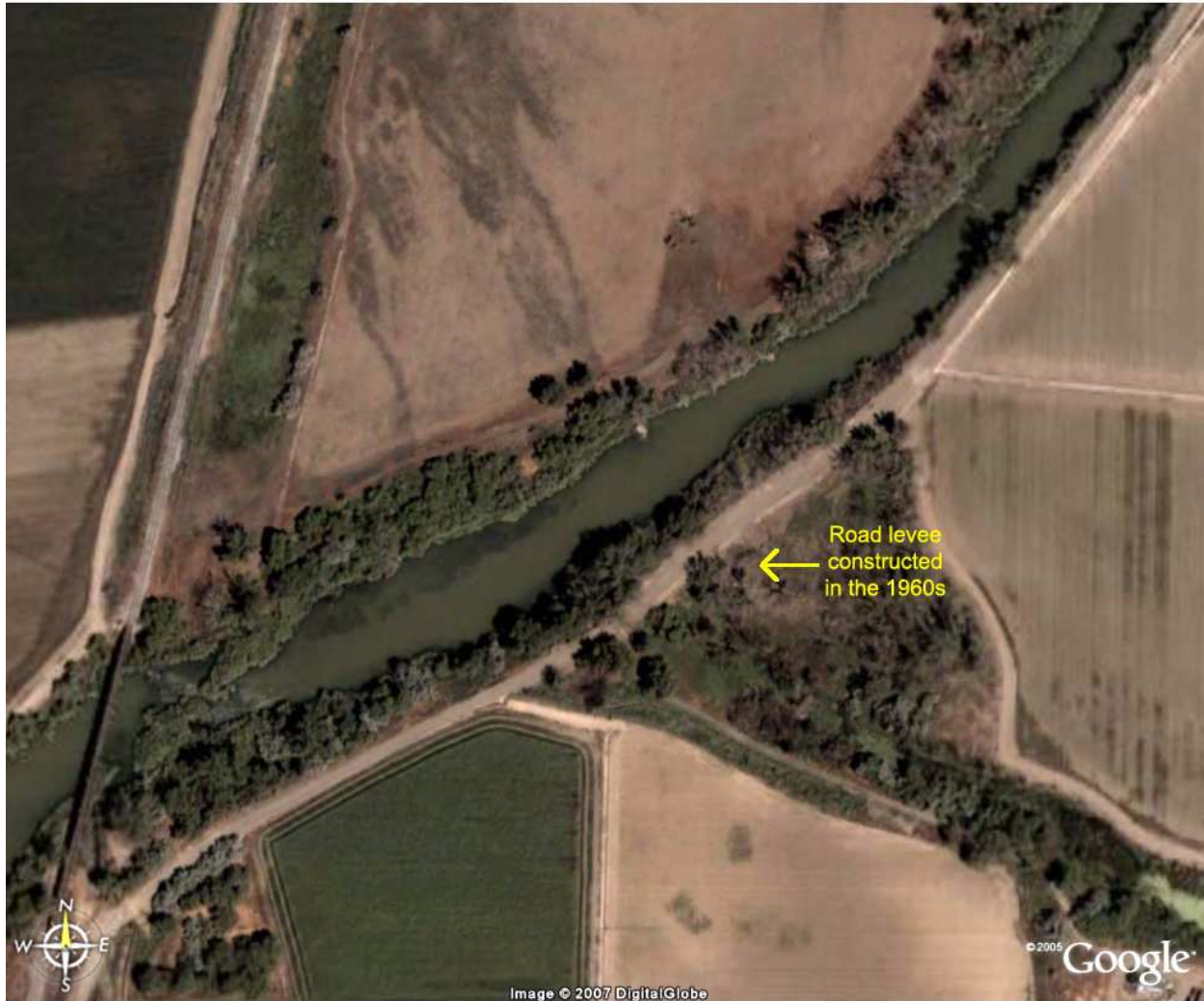
Figure 12.3. Aerial view of the road construction which cut off water flow into the old Owyhee slough.
