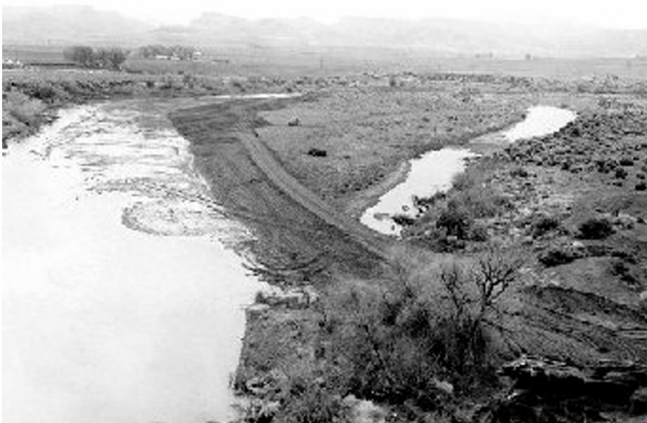
A berm and access road reconstructed across the entrance to the old Owyhee slough. It washed out repeatedly until the 1960s.
